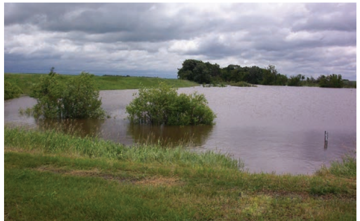
Figure 3: Steppler reservoir with high flood-retention levels (~ 40,000 m 3 ). The water level meter is virtually submerged (lower right of photo).
