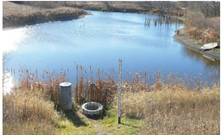
Figure 4: Steppler reservoir with low water levels (~ 4,000-5,000 m 3 ). The water level meter is visible in the foreground.
